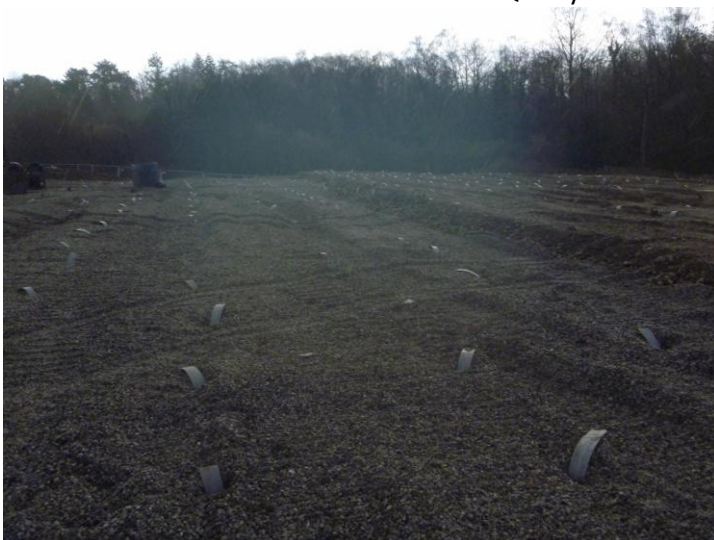
BELOW FIG 1 Vertical Band Drains at Isles Quarry West
