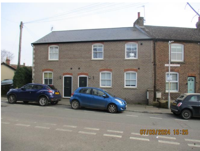
HOADLEYS STORE QUARRY HILL (2 houses)
