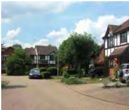
Eaglestone Close and the eastern end of Tolsey Mead are paved.
