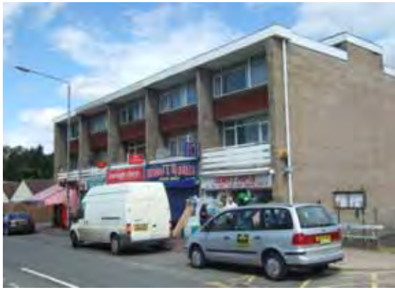
The three/four storey shopping parade is out of character with the village centre in terms of scale, materials and form and is a jarring element in the townscape.
